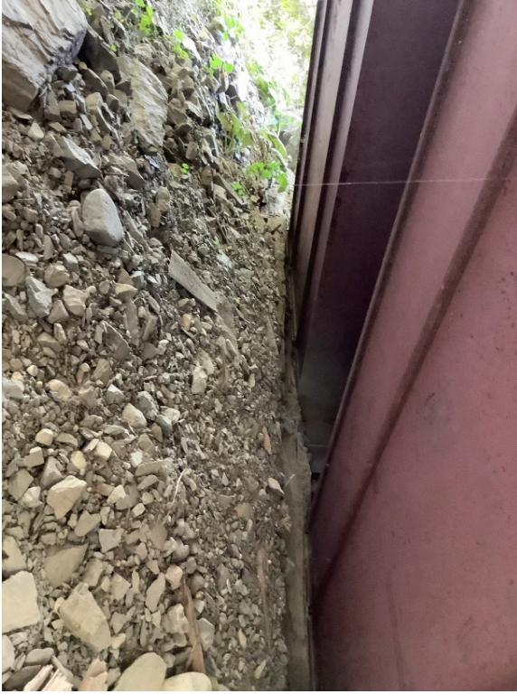
Right Bank Abutment when facing downstream
